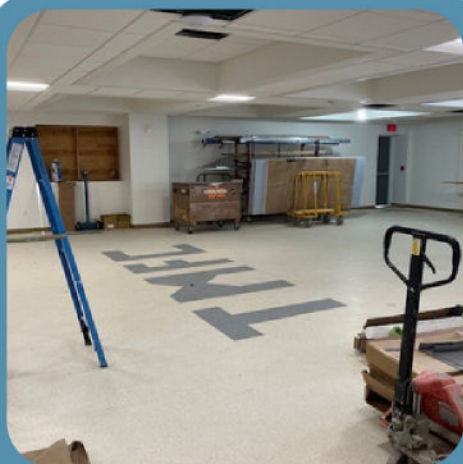
Exciting progress being made during construction at the new location!
